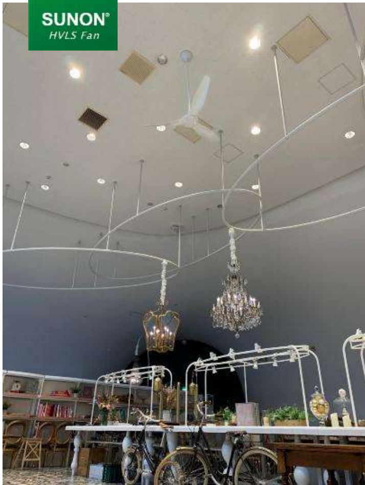
Restaurant of Taiwan Modern HVLS Fan
