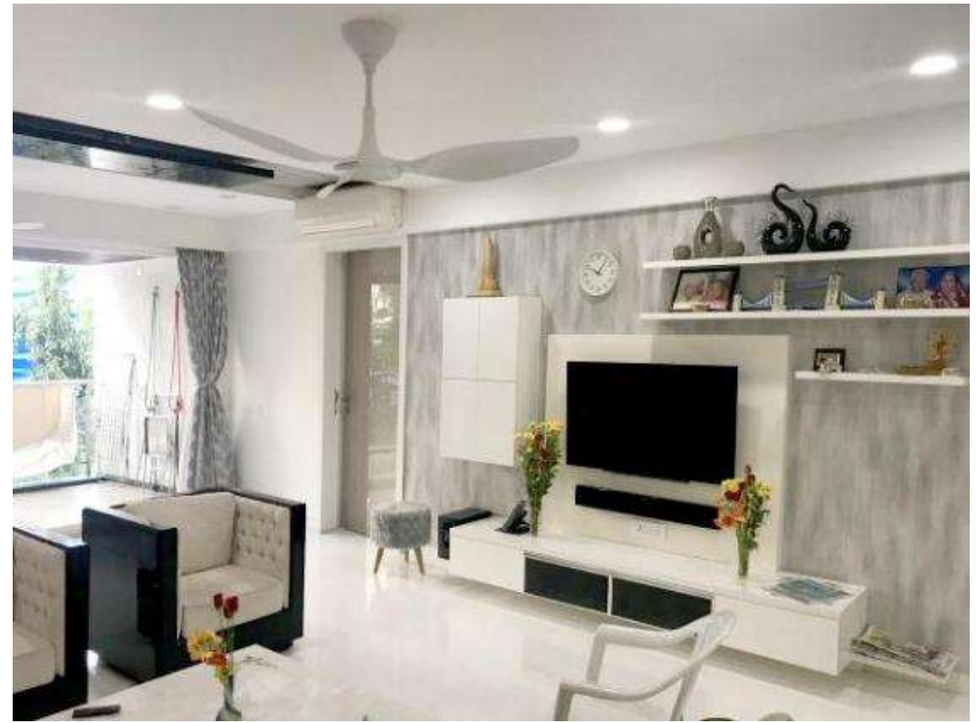
Residential of India Modern HVLS Fan
