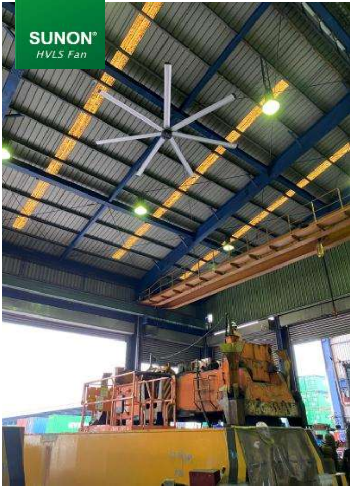
Evergreen Marine Corp. Maintenance Center of Taiwan Series 10
