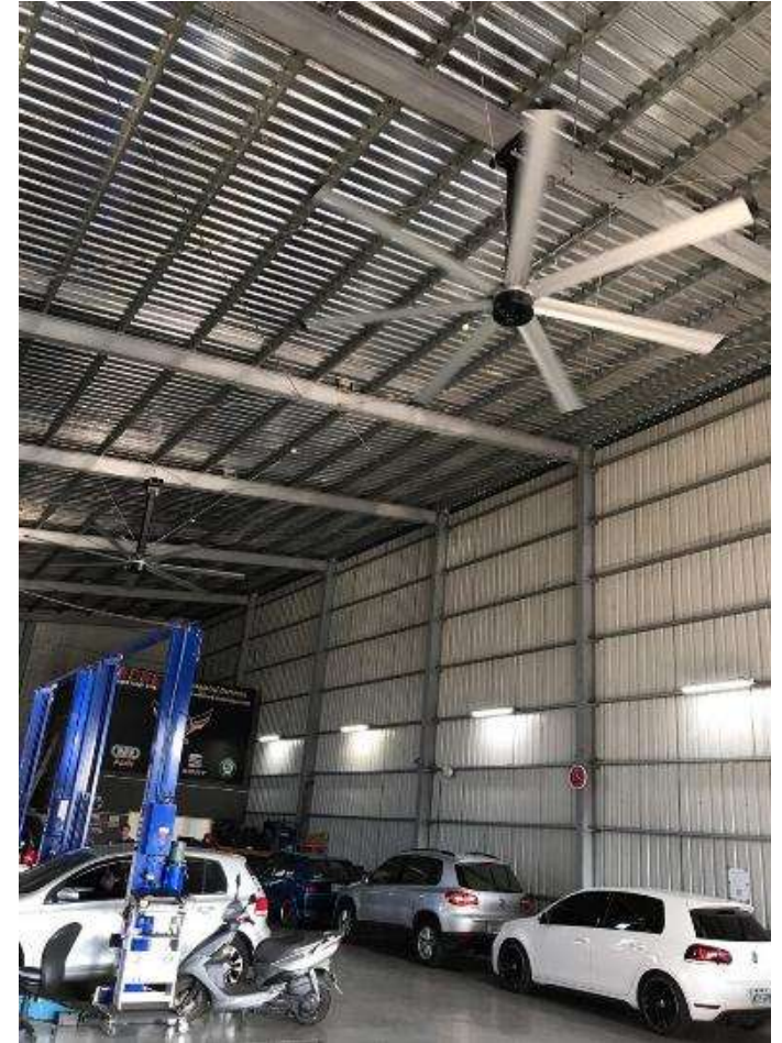
Car Maintenance Center Car Maintenance Center of Taiwan Series 10
